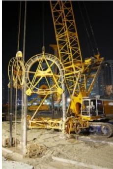
The construction of tunnels can be a hazardous operation. Direct injection of soluble silicates in combination with a hardener, gives consolidation of the ground and water-impermeability by in-situ formation of a siliceous gel, which strengthens and seals the soil.
